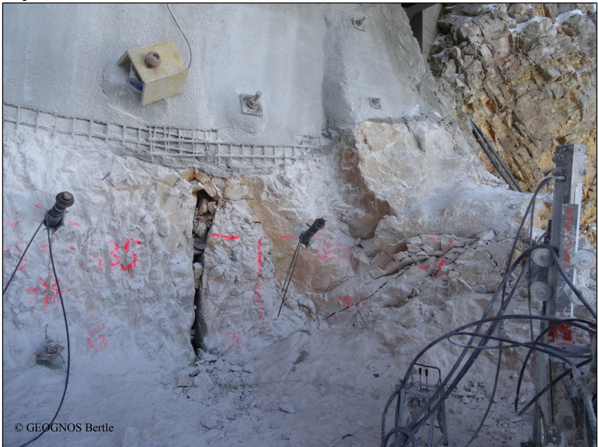
Offene Kluft Baugrube Poller WEST
