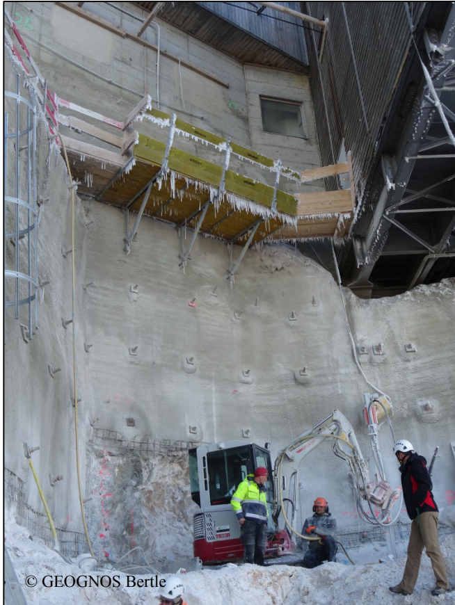
Baugrube Poller West
